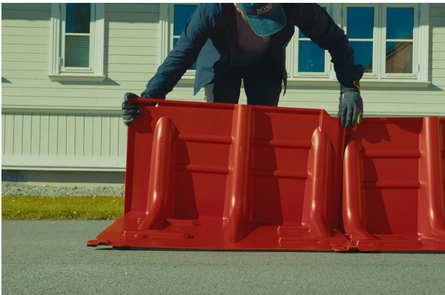
Overlap the heel and press down the rear edge
