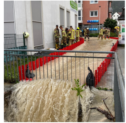
Boxwall as a canal to redirect floodwater through city streets
