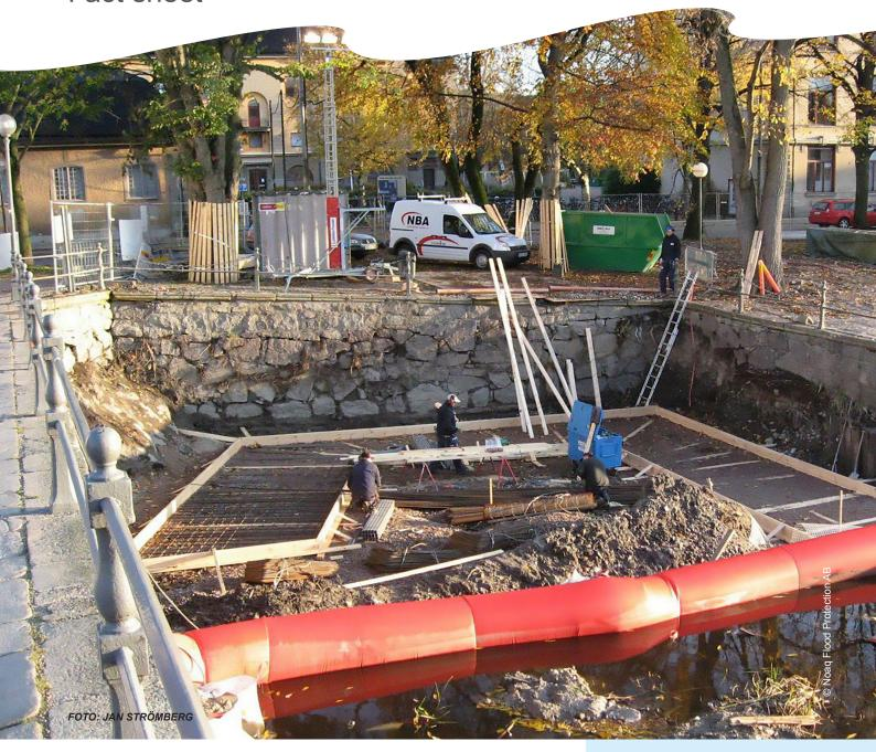
NOAQ Tubewall is a temporary flood barrier. It consists of a number of air inflated sections ("tubes") that are interconnected by ordinary zips to form a continuous protective barrier.
