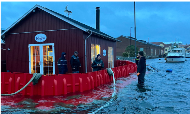
Corners used to provide full perimeter protection
