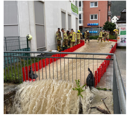
Boxwall as a canal to redirect floodwater through city streets
