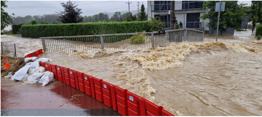
Boxwall diverting and redirecting flashfloods
