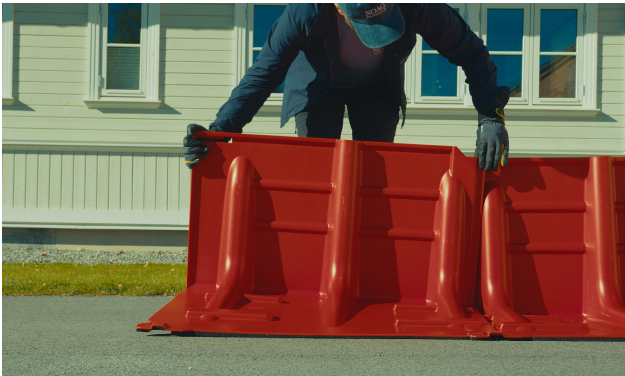
Overlap the heel and press down the rear edge
